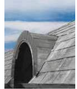
Aspect bardeau zinc
